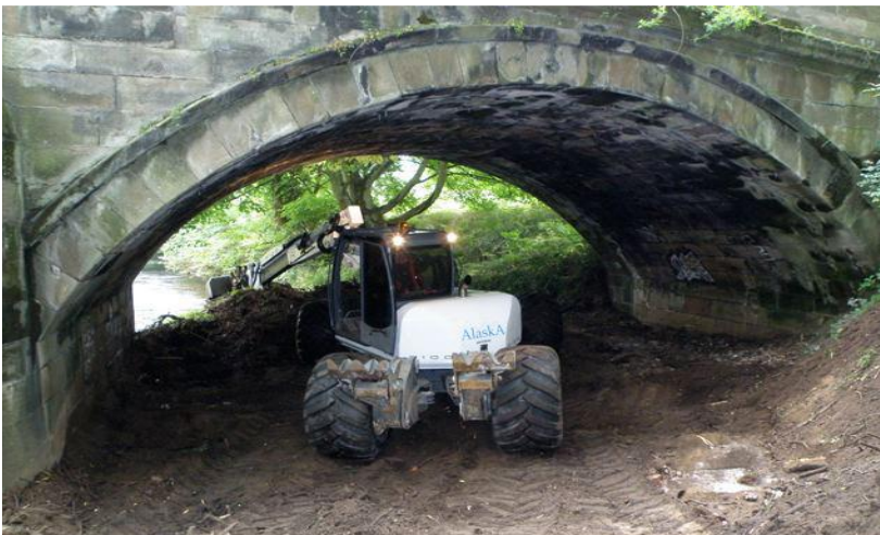
Machine lowered and wheels set in 'narrow' configuration (min width 2.5m)
